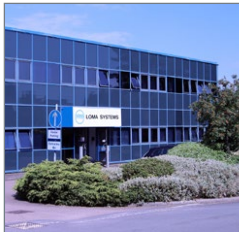
Farnborough, UK - Head Office
